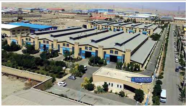
Mechanical Manufacturing Complexes
